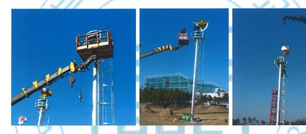
• The wind turbine was installed on the top of the pole. The foundation and installation of the pole and turbine should be considered as important part of a well functioning system. In all cases professionals should handle this process. A good performance can't be guaranteed if the foundation and installation of the pole and turbine are flawed.
